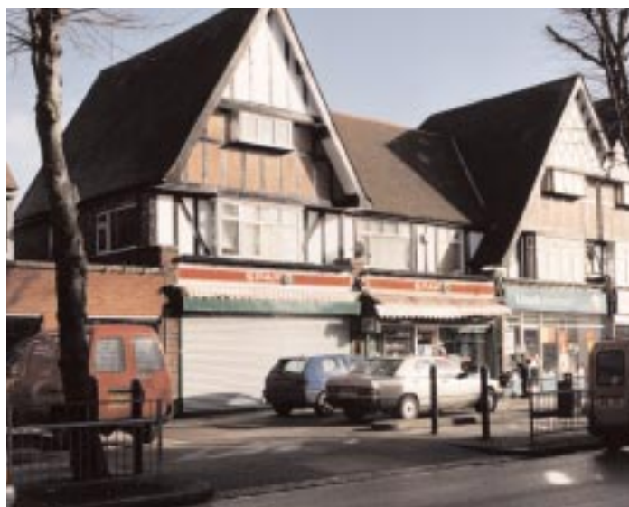
Signage and roller shutters at shops
