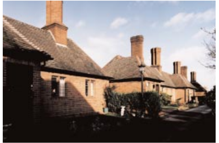
The Charles Lane Trust Almshouses. Rear elevation
