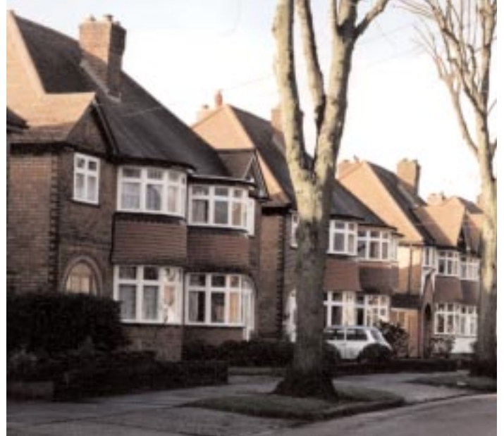
Miall Road ( looking north-west )
