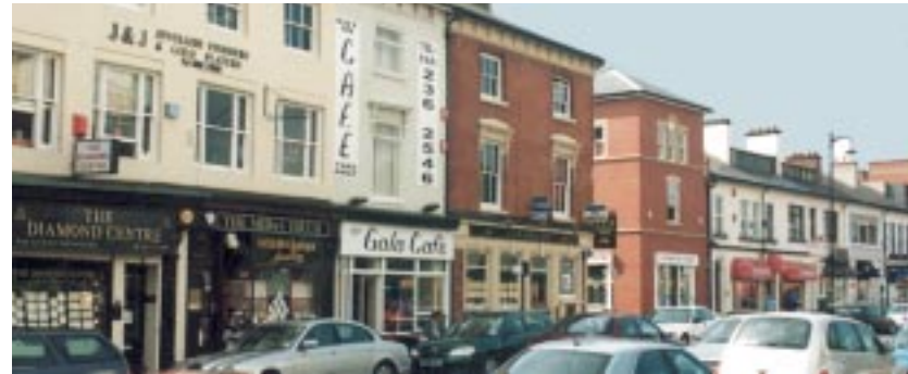
Chimneys adding variety to the roofscape
