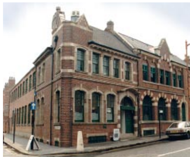
Architectural display on a primary frontage
