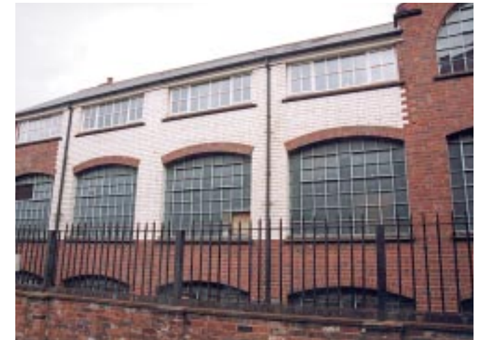
Glazed bricks used to reflect natural light
