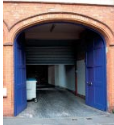
Additional security behind wooden vehicle entrance gates
