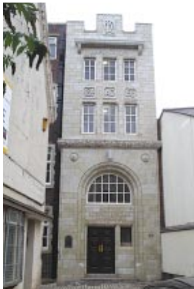
Principal frontage in terracotta
