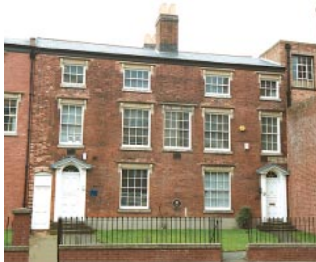
Reinstatement of an historic front plot, boundary walls and railings restored (Birmingham Conservation Trust 1996)
