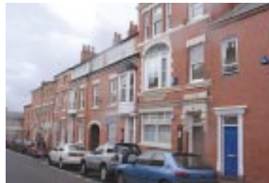
Buildings fronting a secondary street
