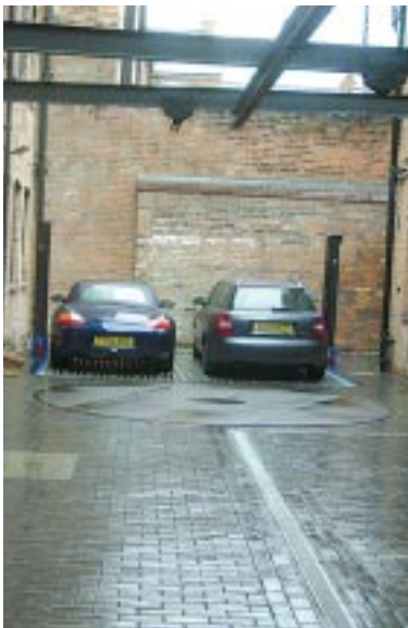
An example of a modern car parking solution in an existing rear yard. A turning plate allows cars to enter and exit in forward gear, and a stacking system enables more cars to be accommodated
