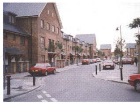
At Chingford Hall, Waltham Forest, on-street parking is part of the adopted roadscape.
