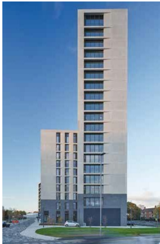
Eastside Locks, Glenn Howells Architects. © Paul Miller.
