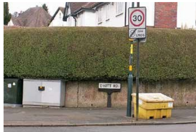
Street clutter Billesley Lane/Dyott Road.
