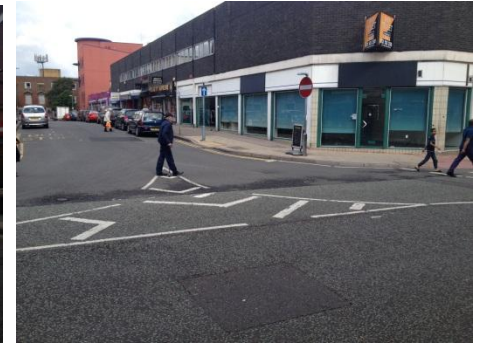
Limited safe crossing points and excessively wide crossing distances present barriers to movement and unnecessarily constrain the available footway widths, impacting on mobility impaired place users in particular.
