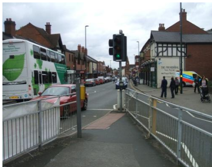
In places the environment is unduly highway dominated. Wide crossing distances and excessive guard railing over-state the link function to the detriment of the place.
