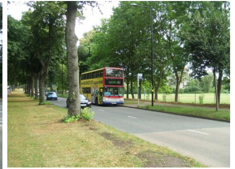
Bus stops lack crossing points. Shared-use cycle paths run along both sides of the road.
