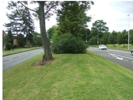
Wide tree lined avenue with three eastbound lanes, including a bus lane (in Borough of Sandwell), and two westbound lanes. Wide grassed central reservation with mature trees throughout.
