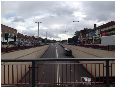
A major A-road (A34) passes through the centre, creating a significant barrier to movement, and carrying large volumes of traffic. Despite being carried via a steep cutting, below street level, traffic noise and emissions are prevalent.
