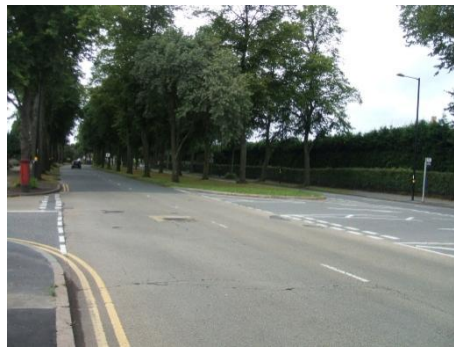
Occasional breaks in the central reservation to facilitate access to side roads. Few crossing points for cyclists and pedestrians along the links.
