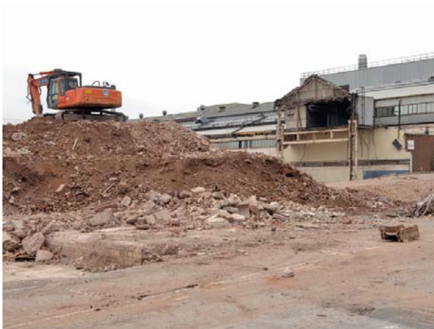
Demolition at Longbridge
