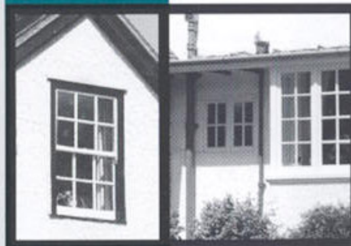
Timber casements with glazing bars
