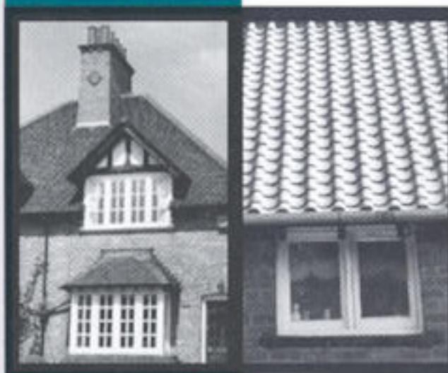
Plain clay tiles have been used on the main roof and on the bay window of this house
