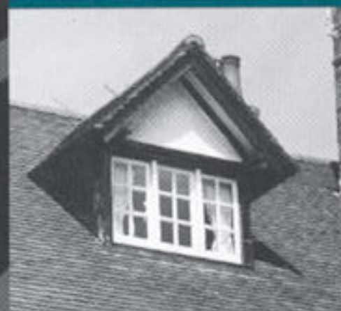
Original flat roofed and gabled dormers are attractive features
