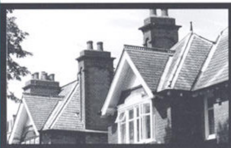
Slate roofs with lead-covered ridges
