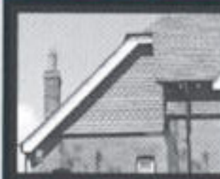
Below Tile hanging
