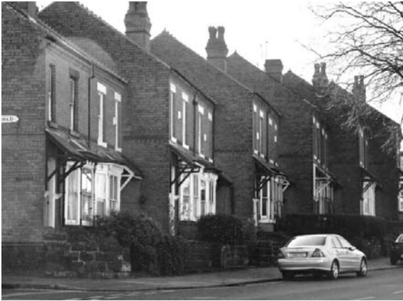
Mid Victorian Cottages: Alcester Road.
